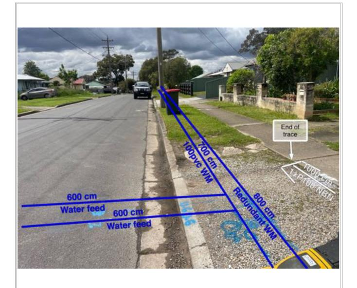
Redundant water main QL-C 100 PVC water main located with GPR, QL-C
