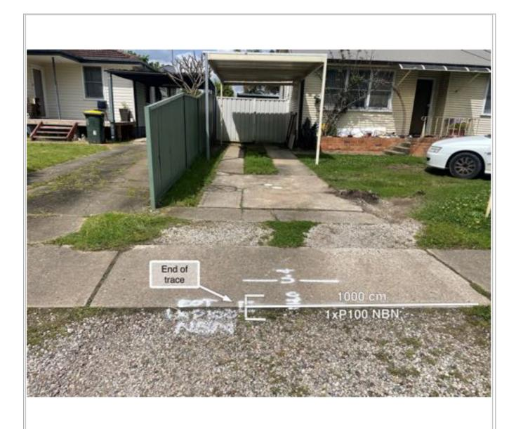
NBN was located QL-B until push rod blocked marked end of trace. From this point was marked QL-D.
