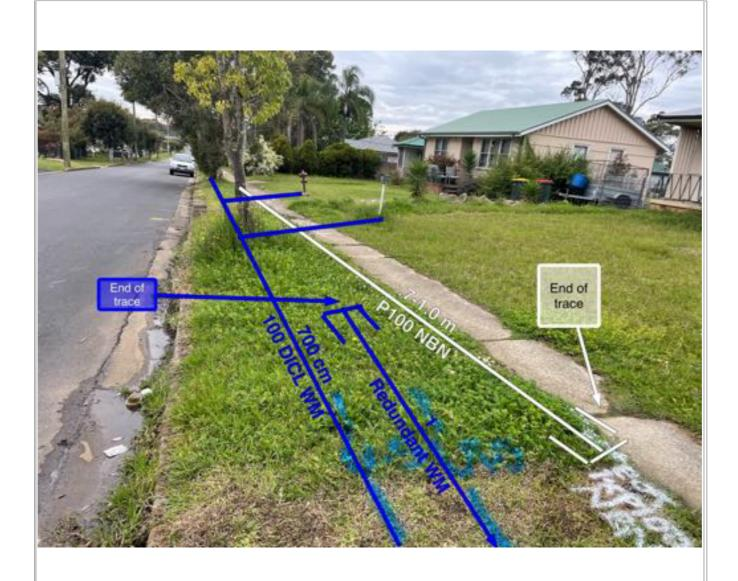
100 DICL Water main, QL-C Redundant water main until loss if signal, QL-C
