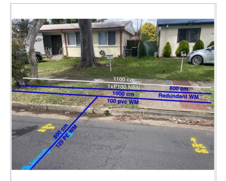
Redundant water main QL-C 100 PVC water main located with GPR, QL-C 125 PE water main located with for, QL-C
