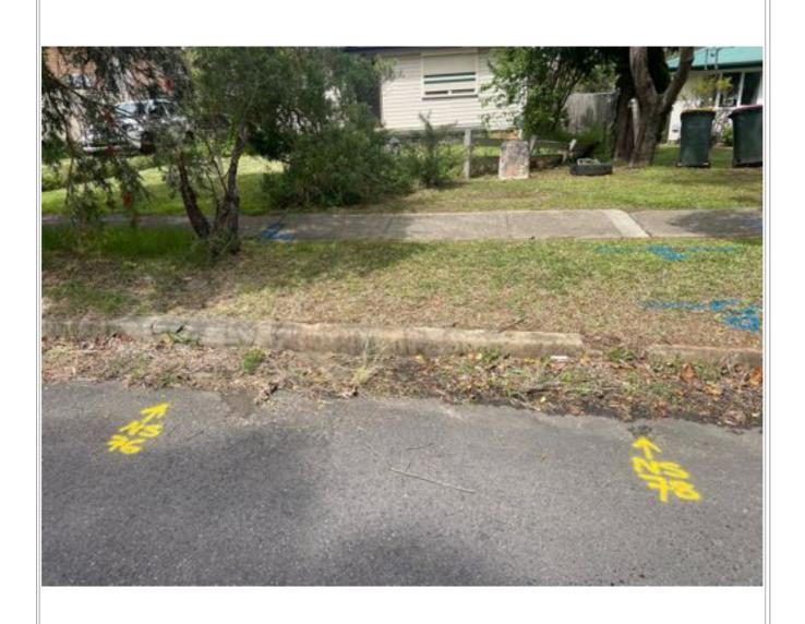
Unable to locate any gas house feeds due to, pipes made from a non-conductive material with no exposed trace wire. Attempted with for but was poor signal due to dense wet clay.
